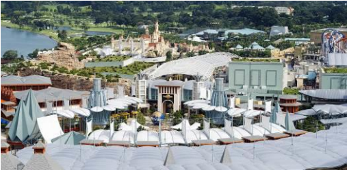
Resorts World Sentosa's ETFE (Ethylene tetrafluoroethylene) roof that keeps its premises cool
